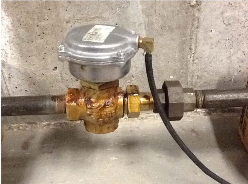
After – DDC control with new thermostat control, balancing and isolation valves
