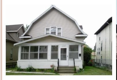
Before: Enclosed front porch was separating from the house. Roof was salvaged, supported, and everything underneath demolished.
