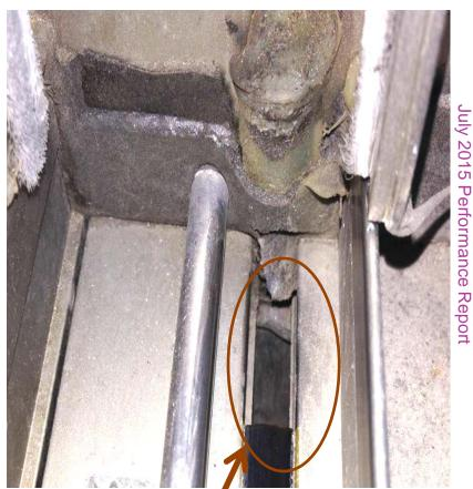
Large hole caused by 'thermal break' shrinkage
