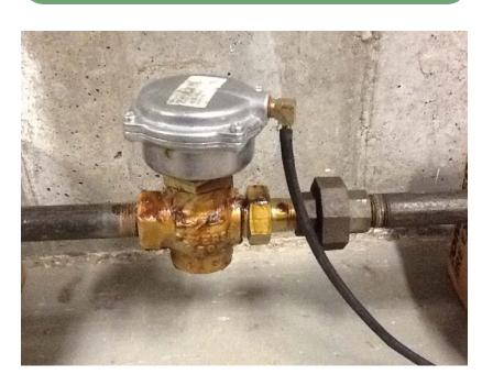
After – DDC control with new thermostat control, balancing and isolation valves
