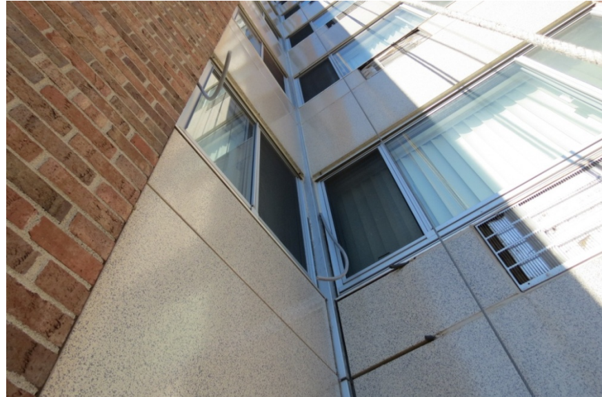
Window perimeter sealant replacement in progress
