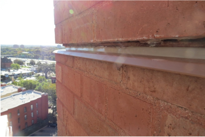
New flashing at horizontal joint
