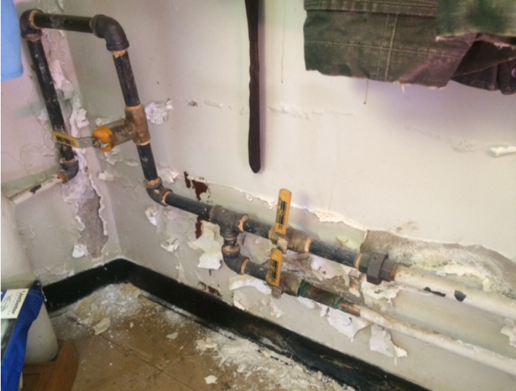
Above: Plaster wall damage in apartments due to hydronic heating system failures
