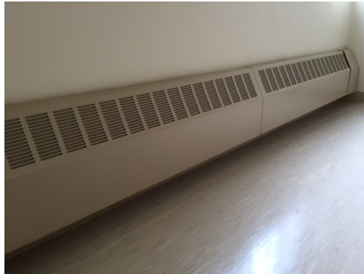
Below: All heating elements replaced with new radiation cover & wall repairs
