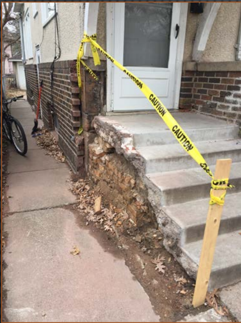
Before: Failed Masonry Stoop
