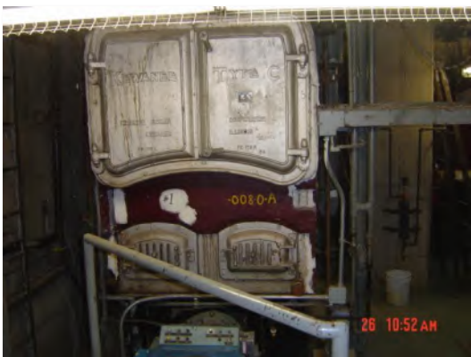
Typical Old High-rise Boiler
