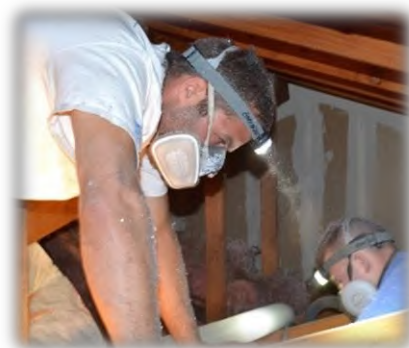
Crews blow in cellulose attic insulation at the Glendale Townhomes.
