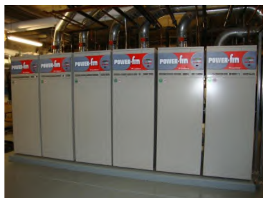
New Boiler Installation
