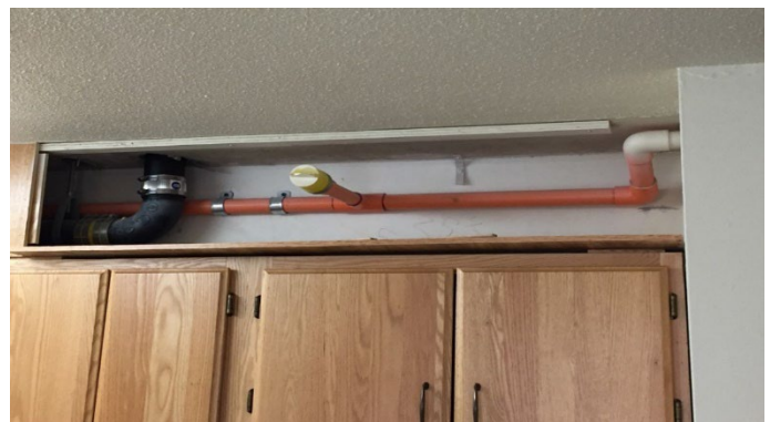
New Fire Sprinklers in an MPHA Unit
